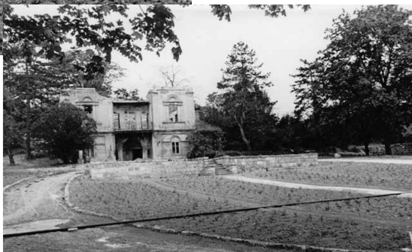
Figure 3: Györgyháza and the Rose Garden under construction
